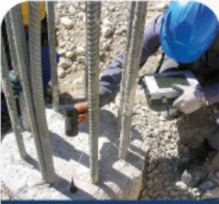
Pile Integrity test
