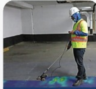
Reinforcement corrosion mapping
