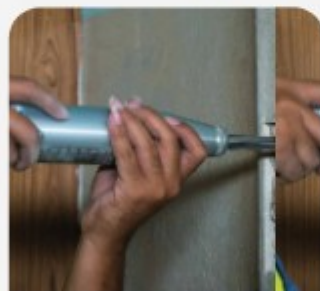
Rebound hammer testing
