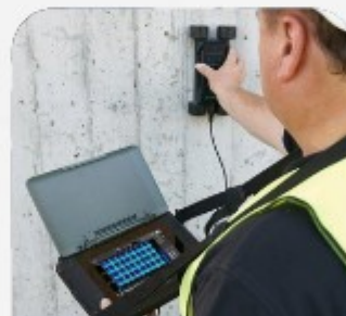
Cover meter testing
