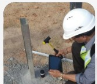
Pile Integrity Testing
